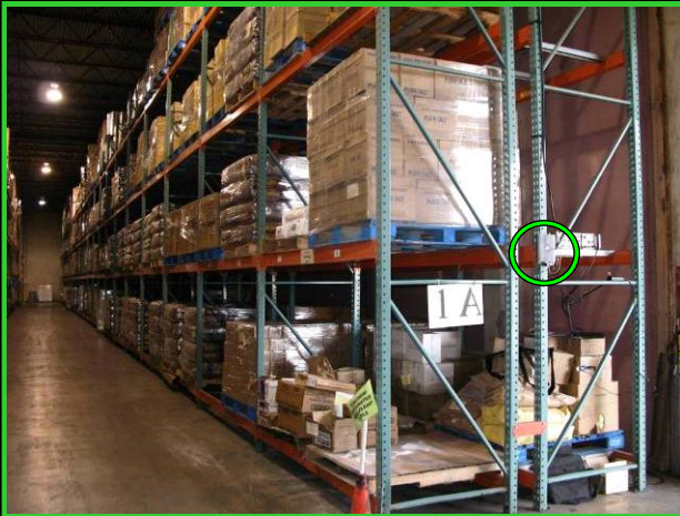
Single Access Point Mounted on Rack
