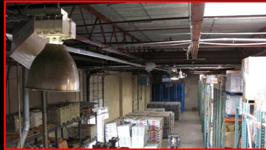
WE Waveguide Along Dock Cross Aisle
